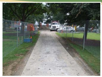
**Special Demolition Procedures** are recommended for demolition of existing sidewalk and curb within CRZs. These measures can vary with the site application. The objective is to protect tree roots under walk and pavement. Such roots may be deep below the base, but some, as in above, may be directly under the paving layer.
