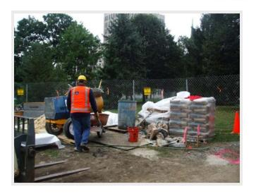
High strength steel fence with signage is specified for installation by the site arborist to protect critical root zones, define equipment access, staging and stockpile, and control "creep" into designated tree protection area.
