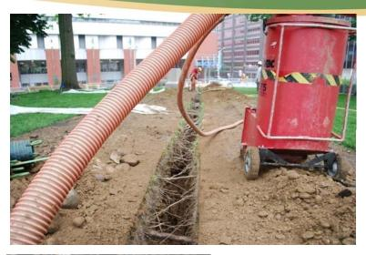
Arborists experienced in high profile construction sites coordinates with the electrician to begin Supersonic Airtool (SSAT) excavation to specified depth for conduits and light pole bases. Note the temporary heavy duty geocomposite matting for root protection during these operations.
