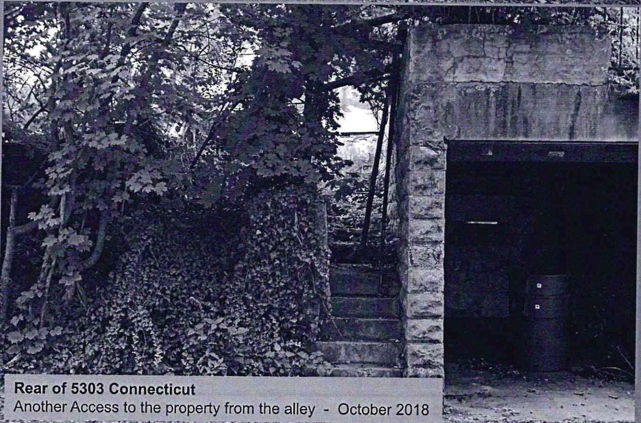
Rear of 5301 Connecticut Easy Access to the site from the alley off Jenifer - October 2018
